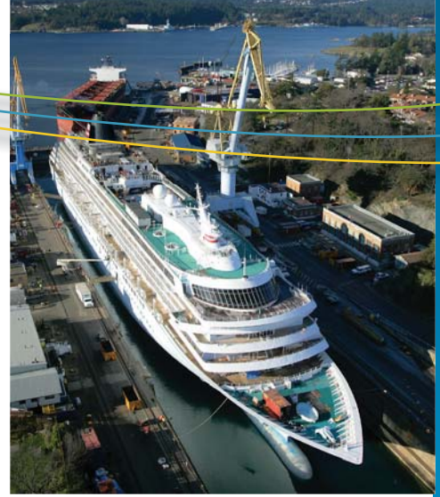
Cruise ship repair services at the Esquimalt Graving Dock
