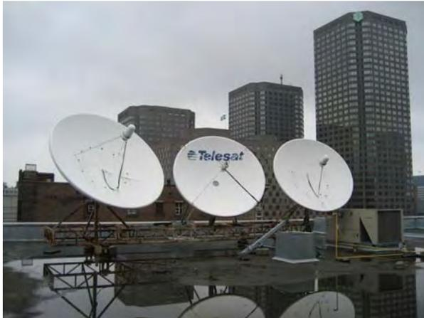
**GTA** (Government Telecommunications Agency) provides a C-Band data service between Ottawa and Iqaluit. It is used to connect government installations in the two capitals. The links operate at data rates of 1536 Kbps and 448 Kbps.
